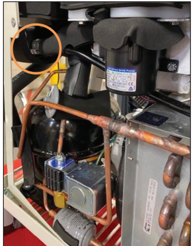
Fig. 8-22 Disconnect two clamps (Step 3- DC pump)
